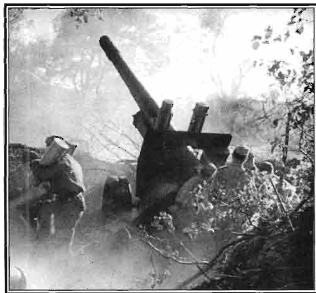
Below: The Soviet barrage caught the Germans by surprise and disrupted their preparations for the offensive. The gun shown below is a Soviet M1937 (ML-20) howitzer firing massive 152mm (6in) shells.
